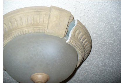
Damaged light fixture in hallway
